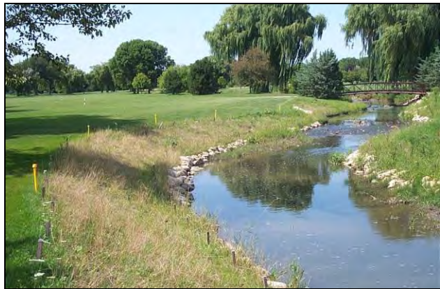
Buffalo Creek Stream Restoration (Source: Baxter & Woodman, Inc.)
