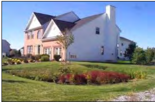
Residential Rain Garden
