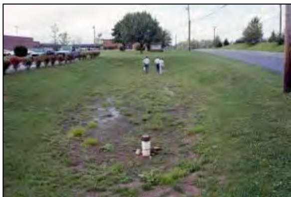
Surface Sand Filter
