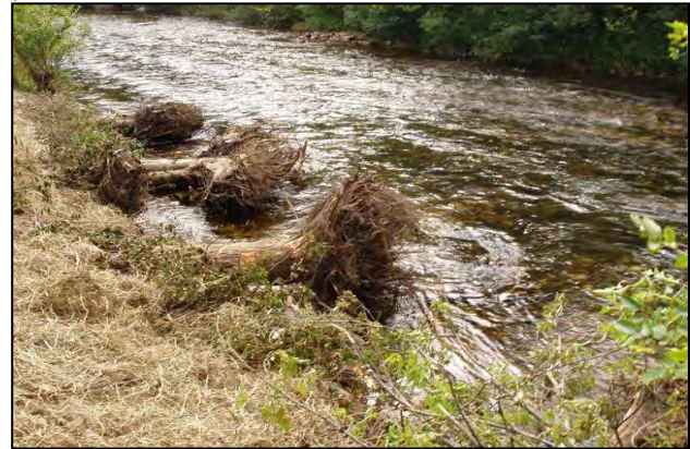
Rootwads to Stabilize a Stream Bank
