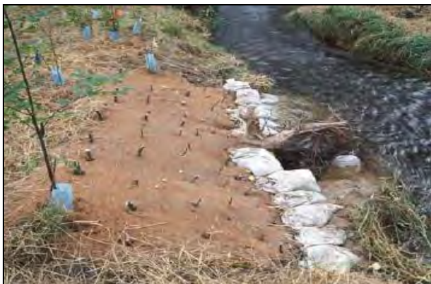
Erosion Control Fabric Along a Streambank (Source: Center for Watershed Protection)
