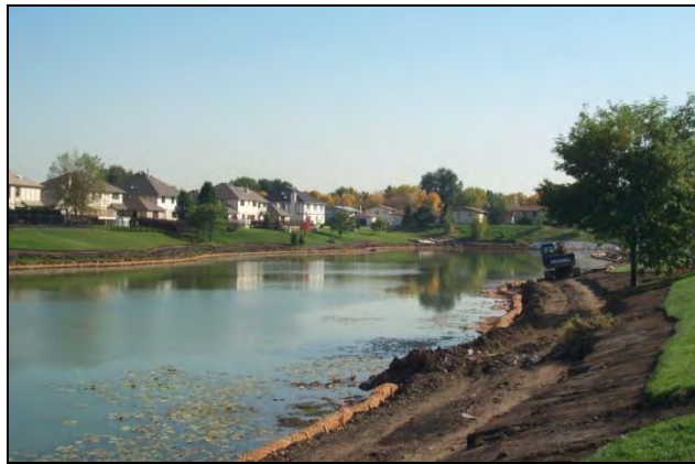
Lake Emily Retrofit, During Construction Oak Forest, IL
