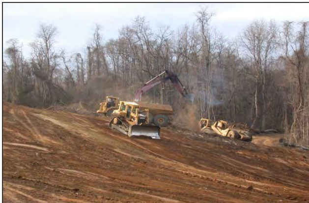
Active Construction Site
