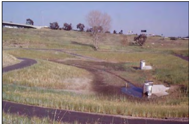
Dry-Bottom Detention Basin
