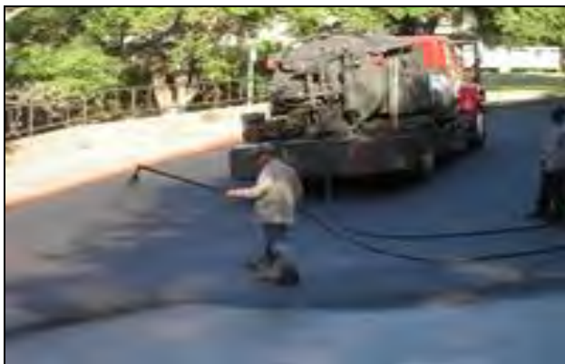
Parking Lot Sealing
