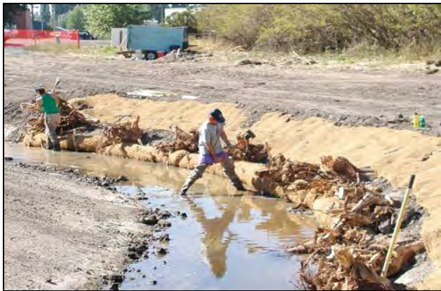
Coir Fiber Logs Along a Streambank (Source: http://www.landandwater.com )
