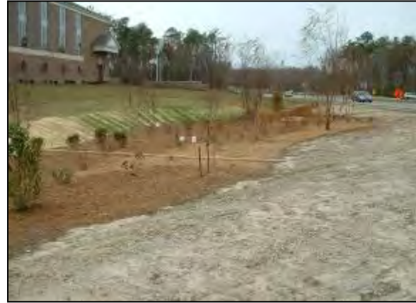
Infiltration Basin (During Installation)
