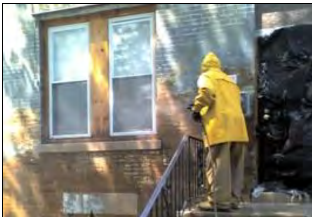
Sandblasting a Single Family Home (Source: http://www.exteriorworldinc.com )
