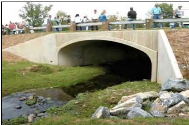
Bridge Installed to Improve Fish Passage
