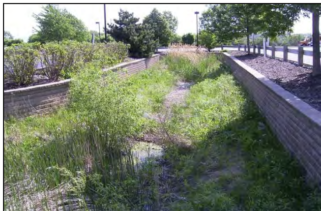
Dry-Bottom Detention Basin in North Barrington
