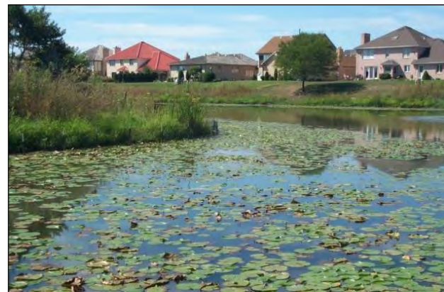
Lake Emily Retrofit, After Construction (Source: Baxter & Woodman, Inc.)
