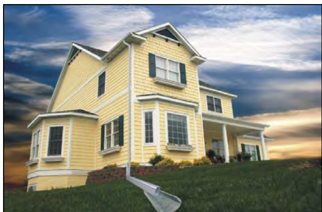
Downspout Disconnection to Lawn (Source: http://www.myhamilton.ca )
