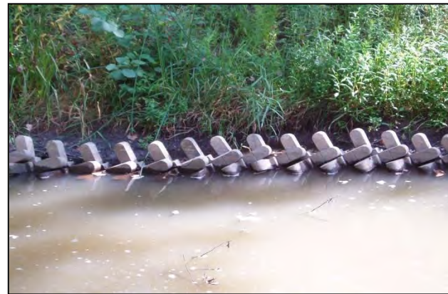
A-Jacks Along the Toe of a Streambank
