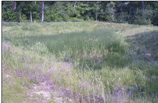
Stormwater Wetland in North Barrington
