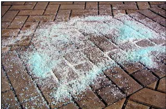
Excess Road Salt on a Driveway
