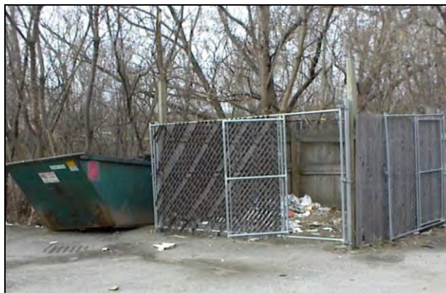
Poor Waste Management
