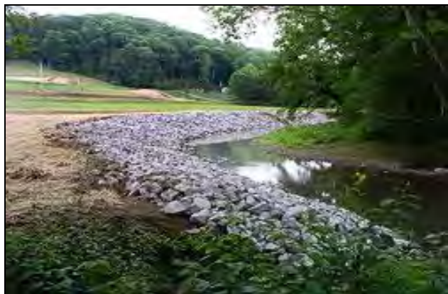
Rip Rap Revetment Along a Streambank
